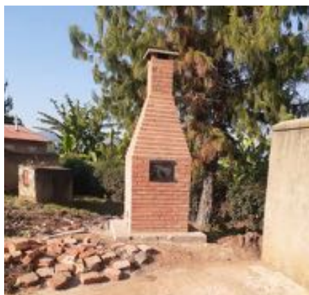
The new incinerator at NGBSS is nearing completion
